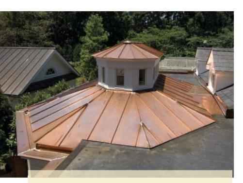
The roof of the conservatory had to be built to properly shed water not only from the new structure but from the roof of the existing two-car garage.
